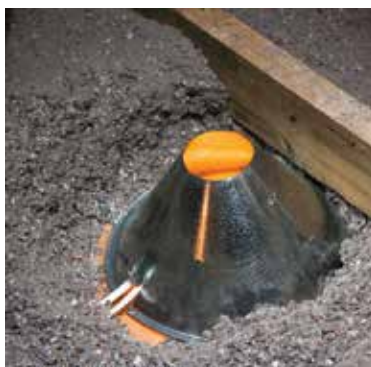
Correct installation of non-combustible cone installed; pre and post-installation. Photos courtesy of Eco Insulation.
