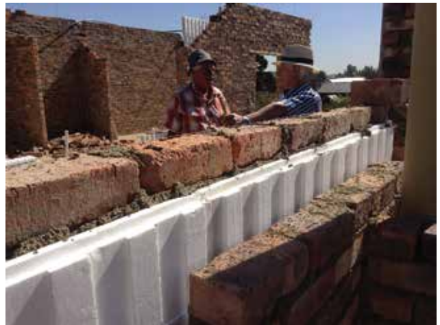
Example of EPS cavity wall insulation. Photo courtesy of Technopol SA (Pty) Ltd.
