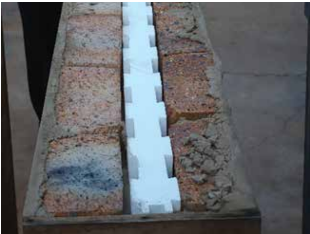
Example of EPS cavity wall insulation. Photo courtesy of Technopol SA (Pty) Ltd.
