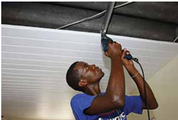
Installation as ceiling and insulation “2 in 1” Photo acknowledgment: Isofoam SA (Pty) Ltd
