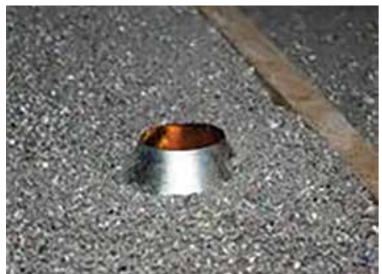
Cellulose blow in fibre can be used in areas difficult to reach. Photographs courtesy of Eco Insulation.
