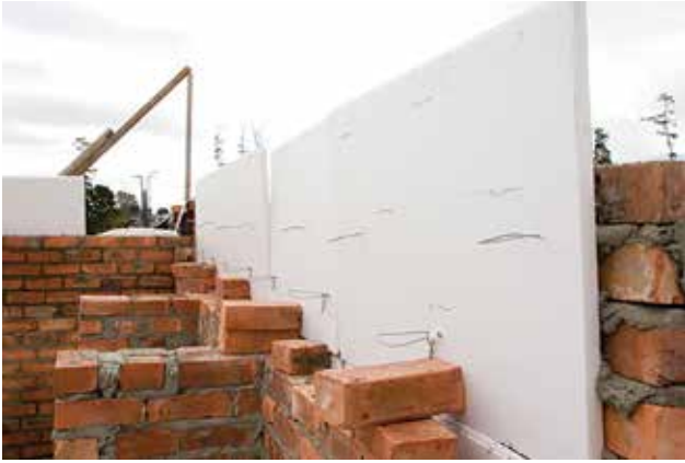
Example of XPS cavity wall insulation. Photo courtesy of Isofoam SA (Pty) Ltd.
