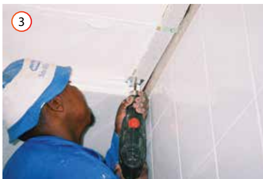
Photo 3: Special clip fixed to existing ceiling
