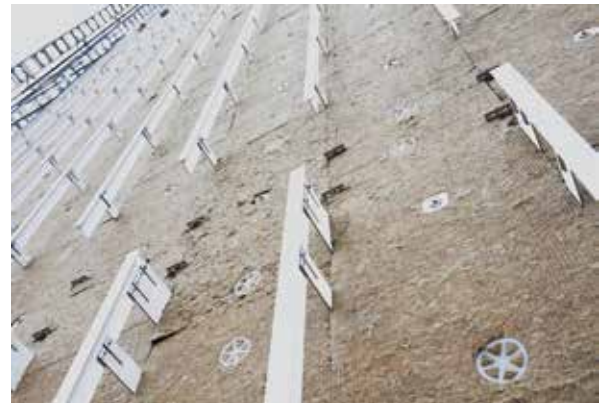
Photograph courtesy of Knauf Insulation Ltd
