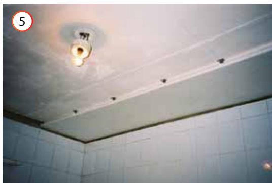
Photo 5: Clips installed and ready for next board to slot in.
