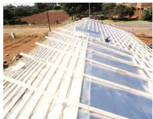
Reflective Foil Insulation/Radiant barrier installed over rafters.
