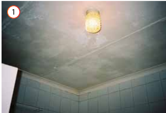
Photo 1: Existing ceiling being prepared.
