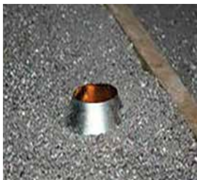
Correct installation of non-combustible cone installed; pre and post-installation. Photos courtesy of Eco Insulation.
