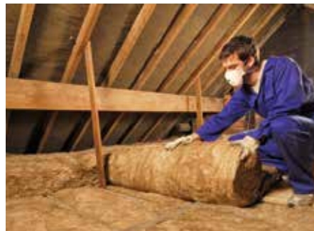
Insulation installed on top of ceiling. Photograph courtesy of Knauf Insulation
