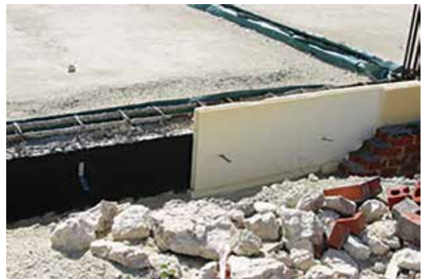
Example of XPS slab on ground insulation and perimeter insulation. Photos courtesy of Isofoam SA (Pty) Ltd.
