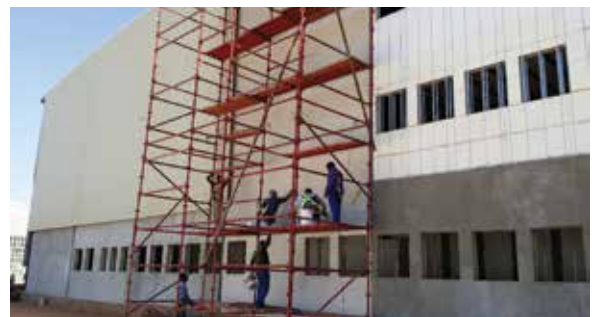
Thermal insulation applied to the external wall and rendered. Photograph courtesy of Technopol SA (Pty) Ltd.
