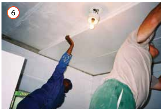
Photo 6: Second board fitted.
