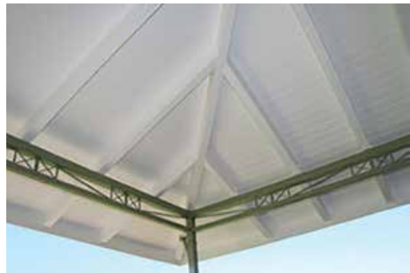
Installation between rafters Photo acknowledgment: Isofoam SA (Pty) Ltd
