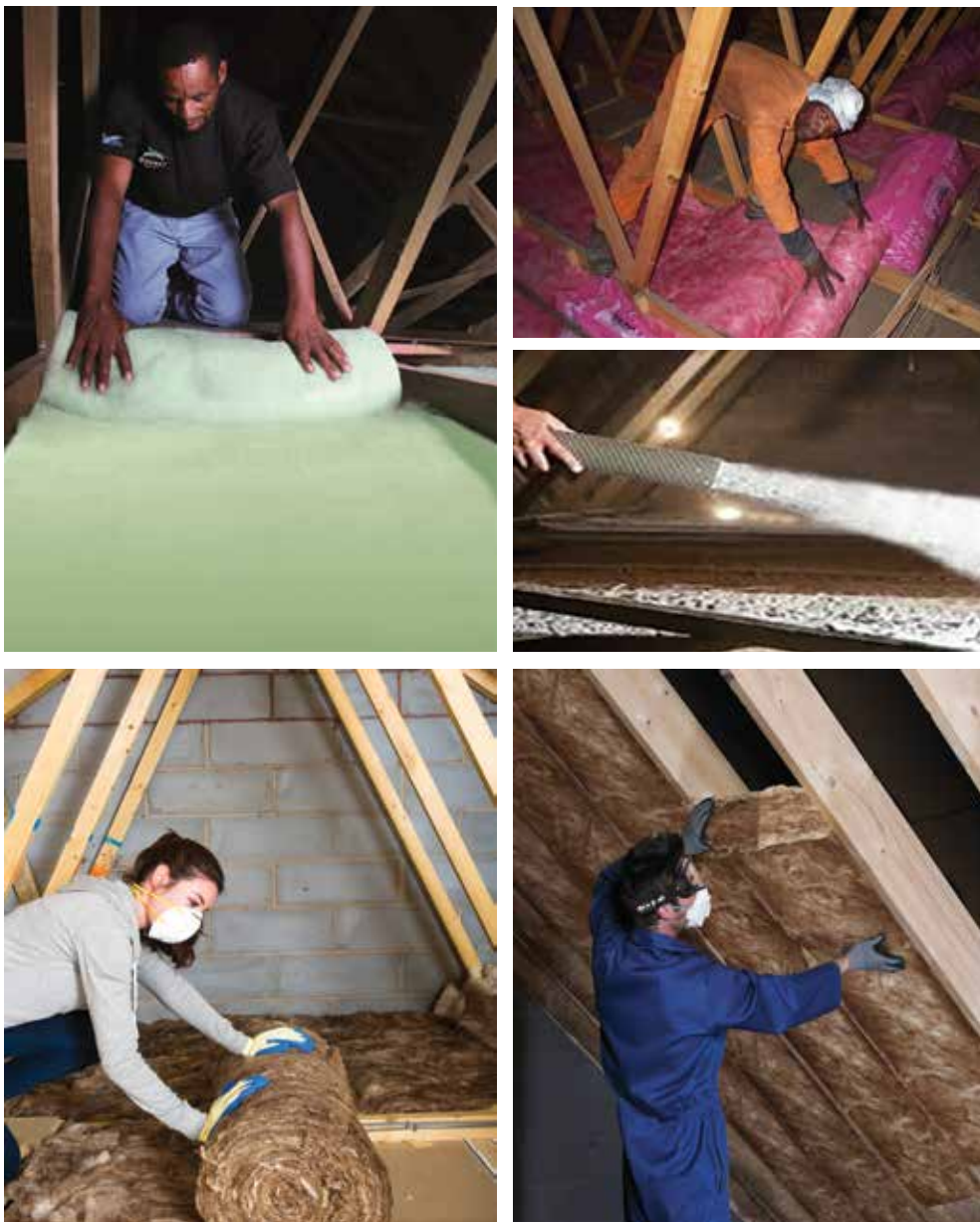
Retrofitting thermal insulation in the ceiling area is an easy energy efficient intervention method.
