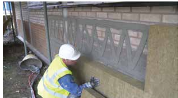
External wall insulation system.
