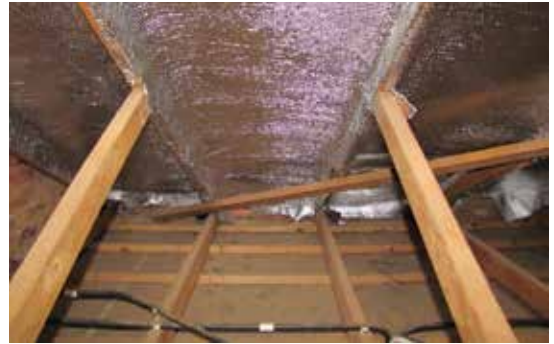
Reflective Foil Insulation retrofitted under roof. Photograph courtesy of Africa Thermal Insulations.
