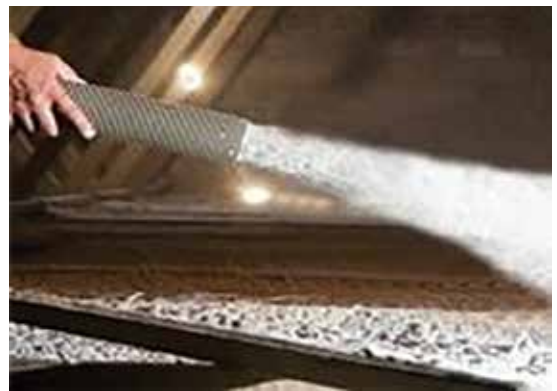
Cellulose blow in fibre can be used in areas difficult to reach. Photographs courtesy of Eco Insulation.
