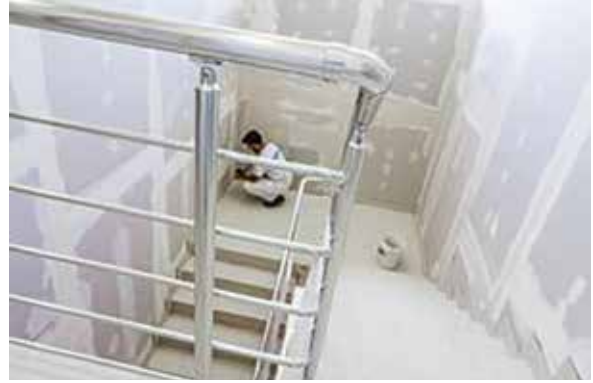
Drywall frame work.
